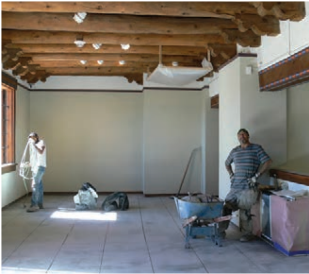
Workers from Advanced Concrete Design in the Beauregard Gallery, after they removed the initial layer from the floors with a terrazzo grinder. Photograph by Michelle Gallagher Roberts.
