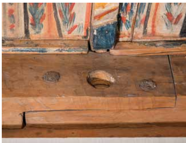
Evidence in the altar screen baseboard of the missing central crucifix.
