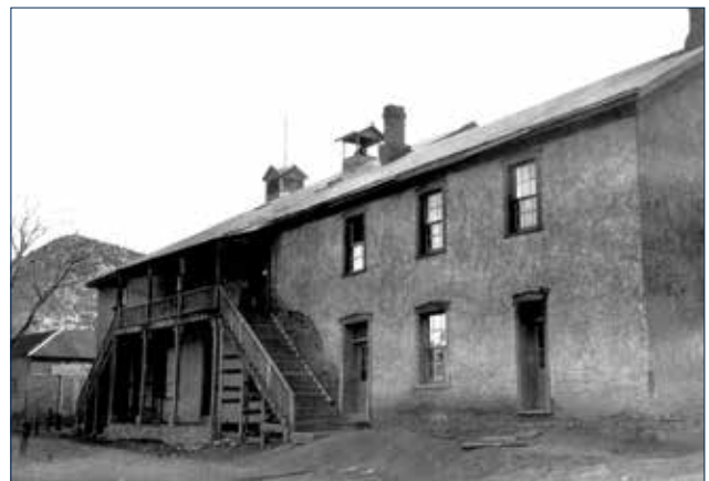
The courthouse in the 1920s, when it was used as a school.
