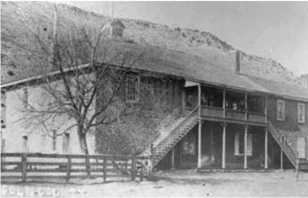
The restored courthouse , ca. 1940. Photographer unknown. Phillip J. Rasch Collection, Lincoln Historic Site.
