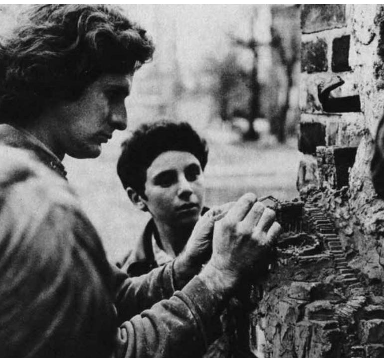
Simonds constructing Dwelling Kreuzeberg in Berlin in 1978.
